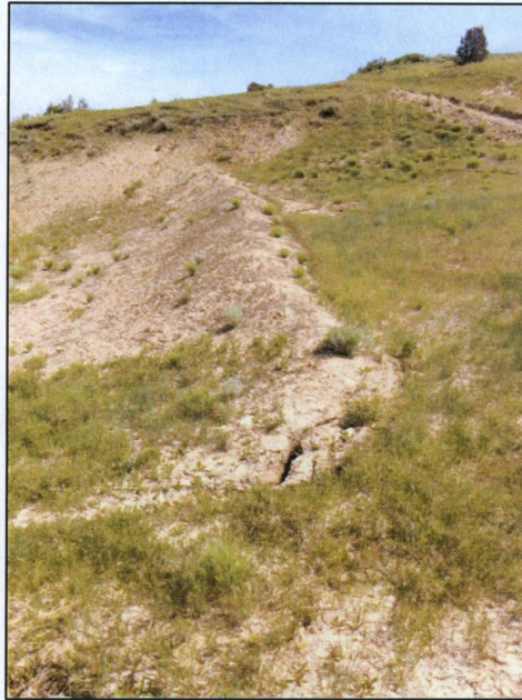
Photograph 5. Upper berm area. View to north
